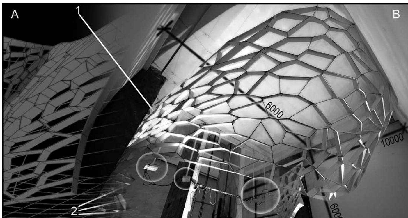
Figure 6 [A] Fragment of the locally variable Voronoi-cell structure conforming to the shape of the dynamic surface (digital rendering). [B] The outer shell in construction on site (photograph). <1> Disused lift shaft. <2> Video projectors.
