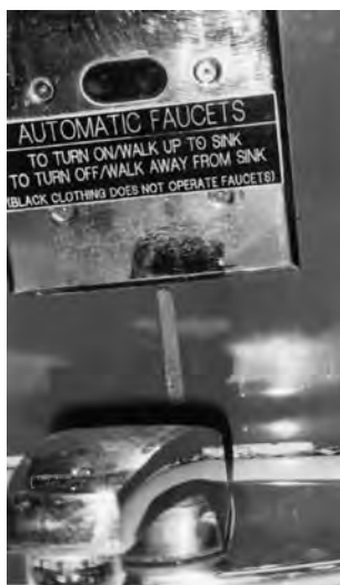
Figure 1 Sensor-based taps in the restrooms at Cincinnati airport.
